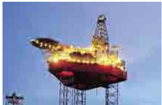
The West Callisto jackup rig is powered by Cat 3516BHD and 4508B engines
